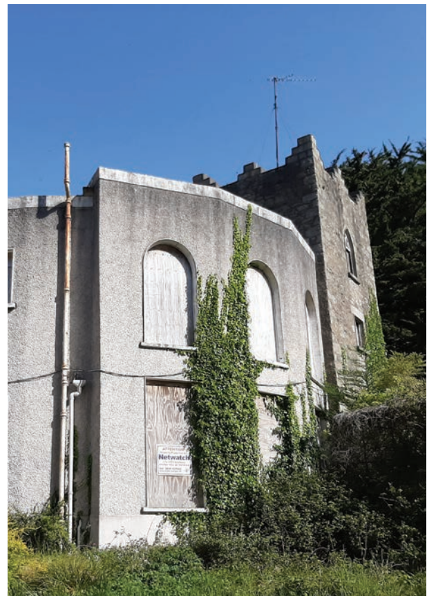
View of the house and tower from the south-east
