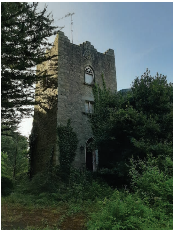
View of the tower from the north-west
