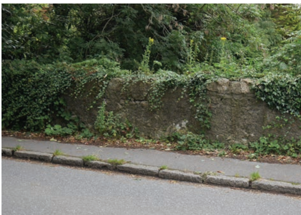
Existing stone wall on the northern side of Brennanstown Road
