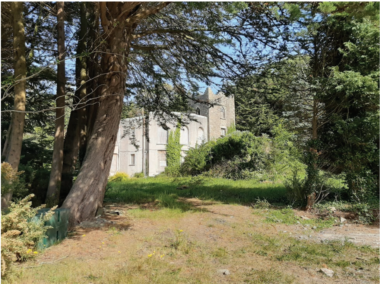
View of the house and tower from the south-east
