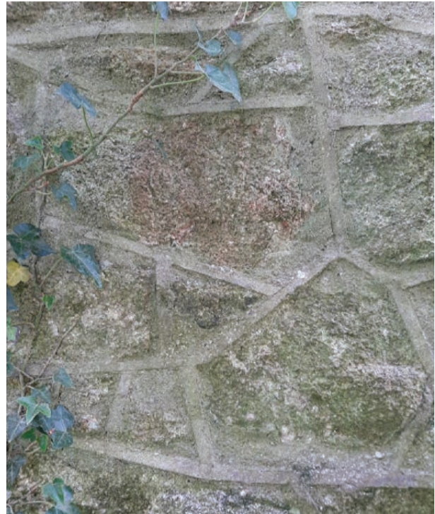
Cement strap pointing to the external walls
