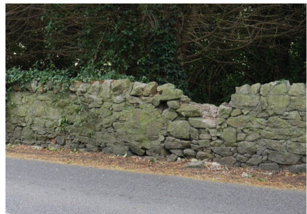
Existing stone wall on the southern side of Brennanstown Road
